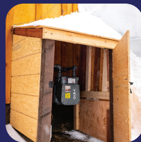
METER WITH SNOW SHELTER
